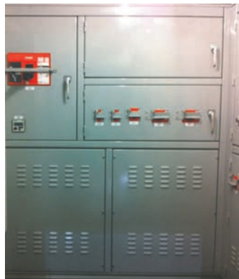
Modular design expandable with multiple VFDs via common DC bus
