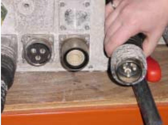
Fig 14: P5 Inverter after Salt Test
